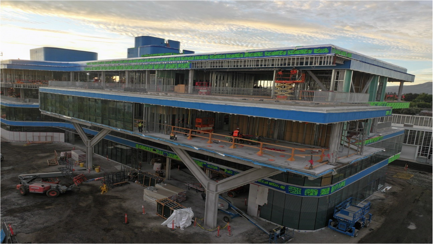
Level 3 Glazing Installation
