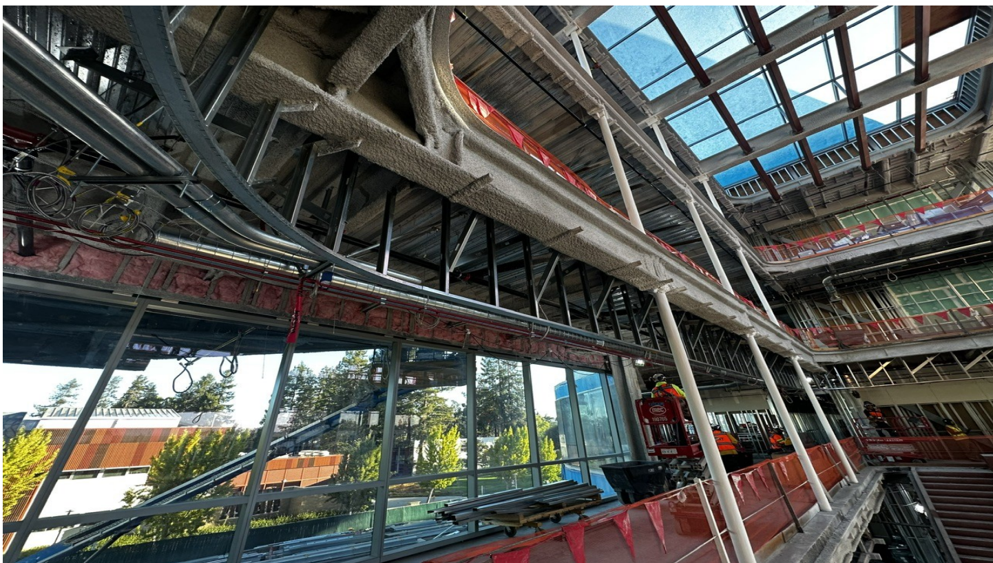
Level 2 Atrium Soffit Framing
