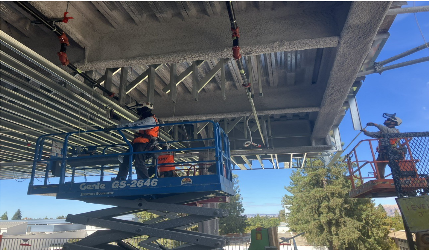
Level 3 Exterior Ceiling Framing
