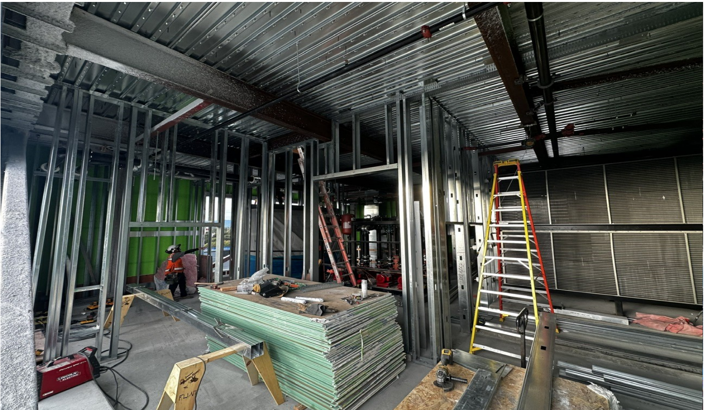
West Penthouse Interior Framing
