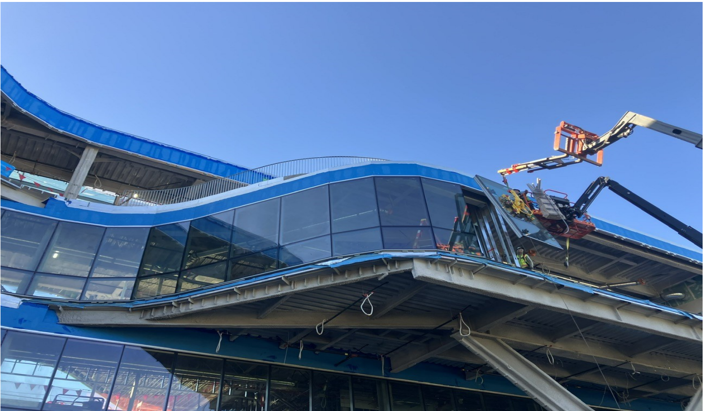
Level 3 Glazing Installation
